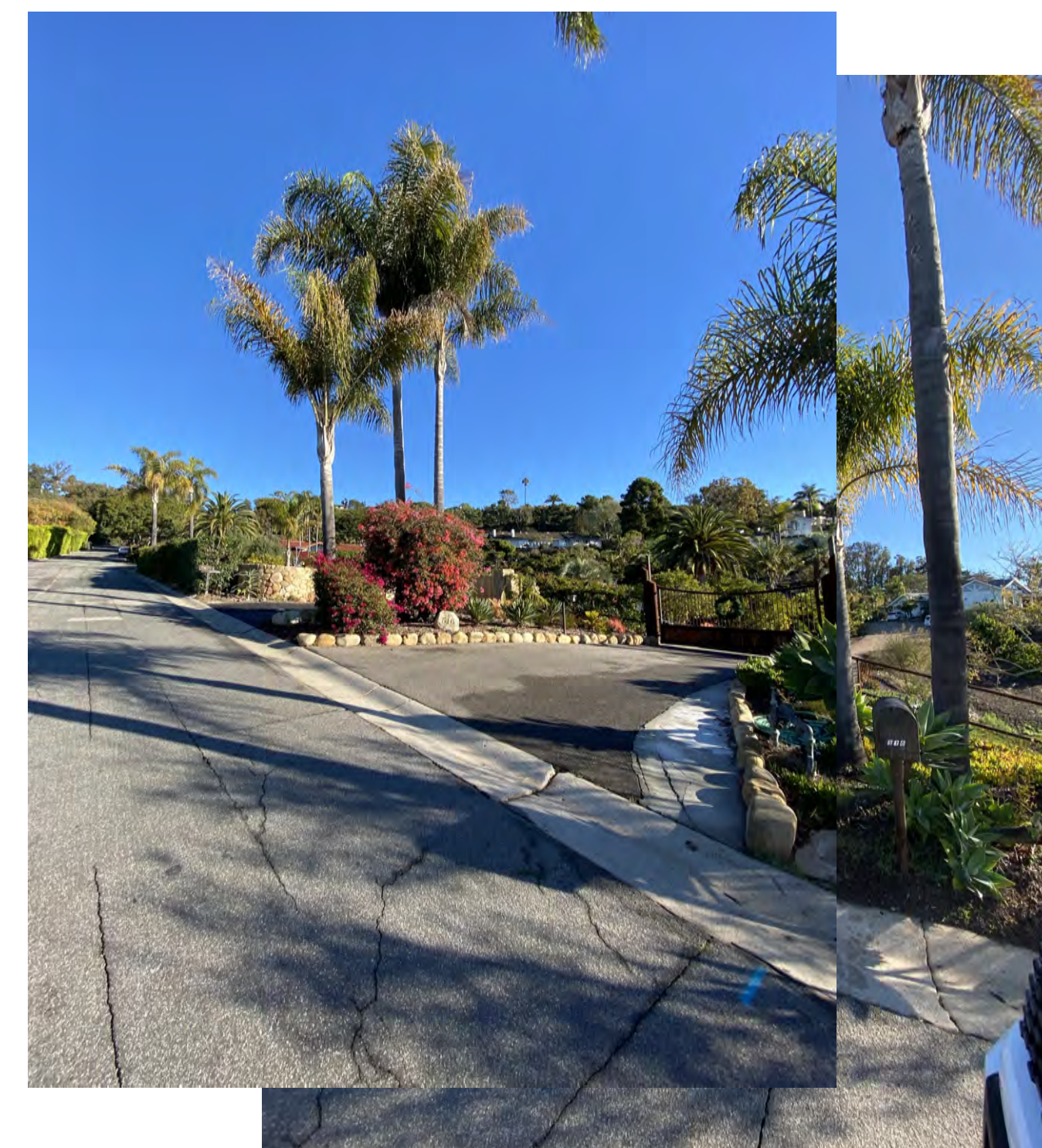
8 DRIVEWAY ENTRY GATE
