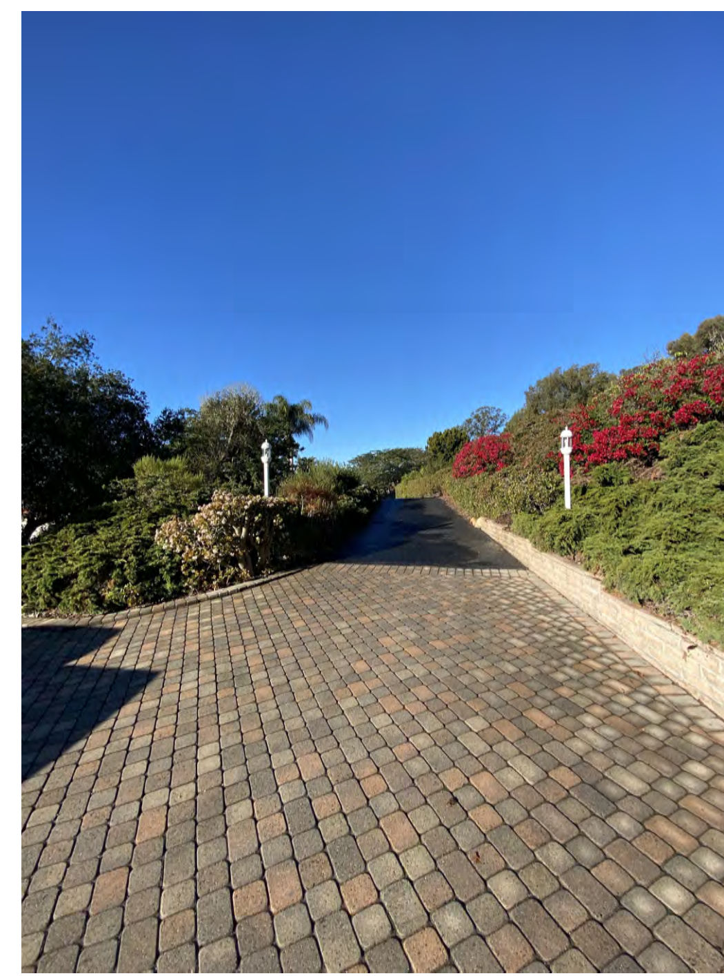
10 DRIVEWAY LOOKING WEST
