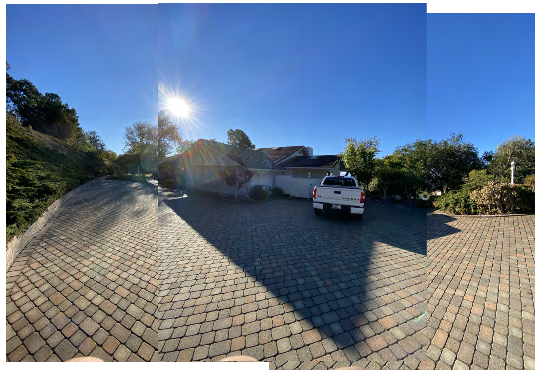
6 FRONT OF RESIDENCE/ NORTH ELEVATION
